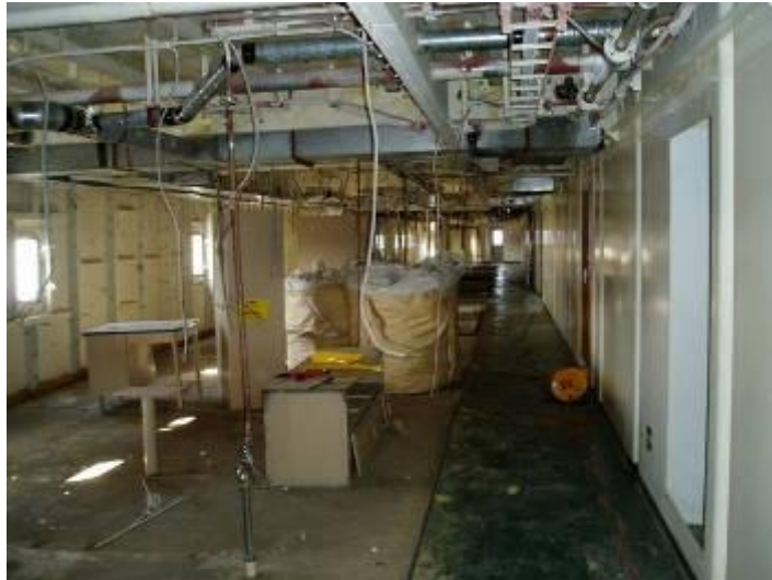
Remove insulating material manually
